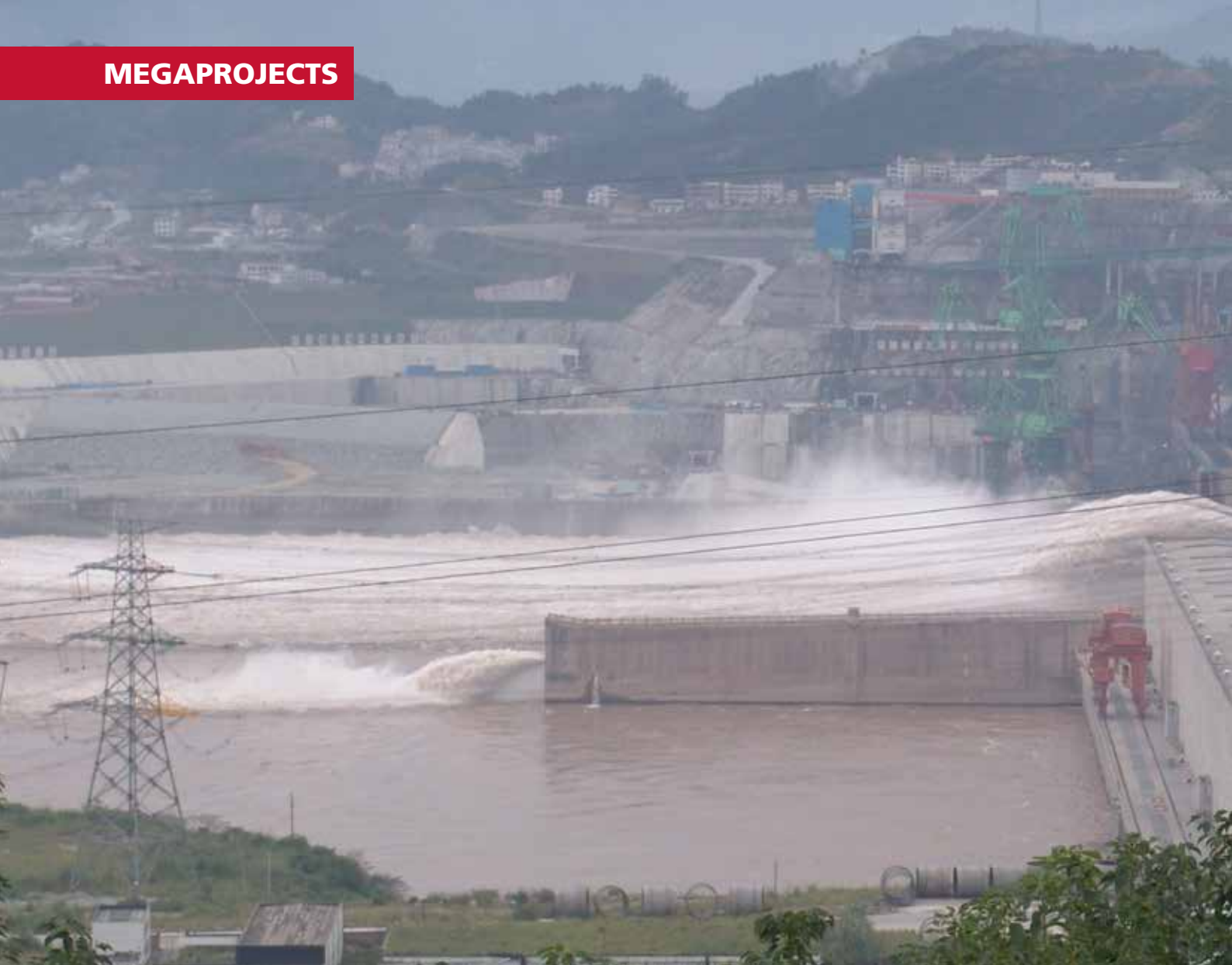
The Three Gorges Dam in China – the world's largest power station in terms of installed capacity (22,500 MW). Credit: Thomas Barrat / Shutterstock
